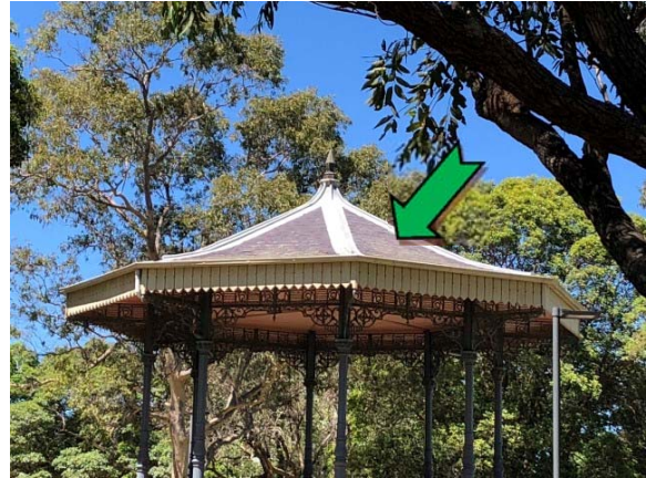
Photo 2. Exterior, throughout, roof – suspected non asbestos-containing roof tiles.
