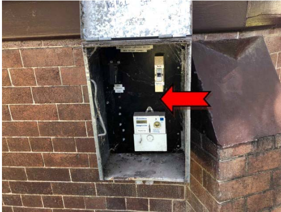
Photo 1. Exterior, electrical backing board – suspected asbestos-containing bituminous backing board.
